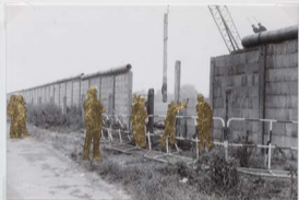
DESTROYED WALL RECONSTRUCTED - 14.07.1973
