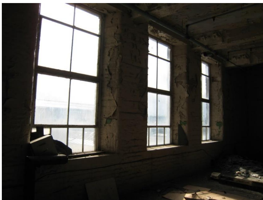
4.15 Quarini, C. Photograph taken on my first research visit to Salts Mill in 2011, showing a disused area with peeling paint and broken windows, used as inspiration. Photo: C Quarini.
