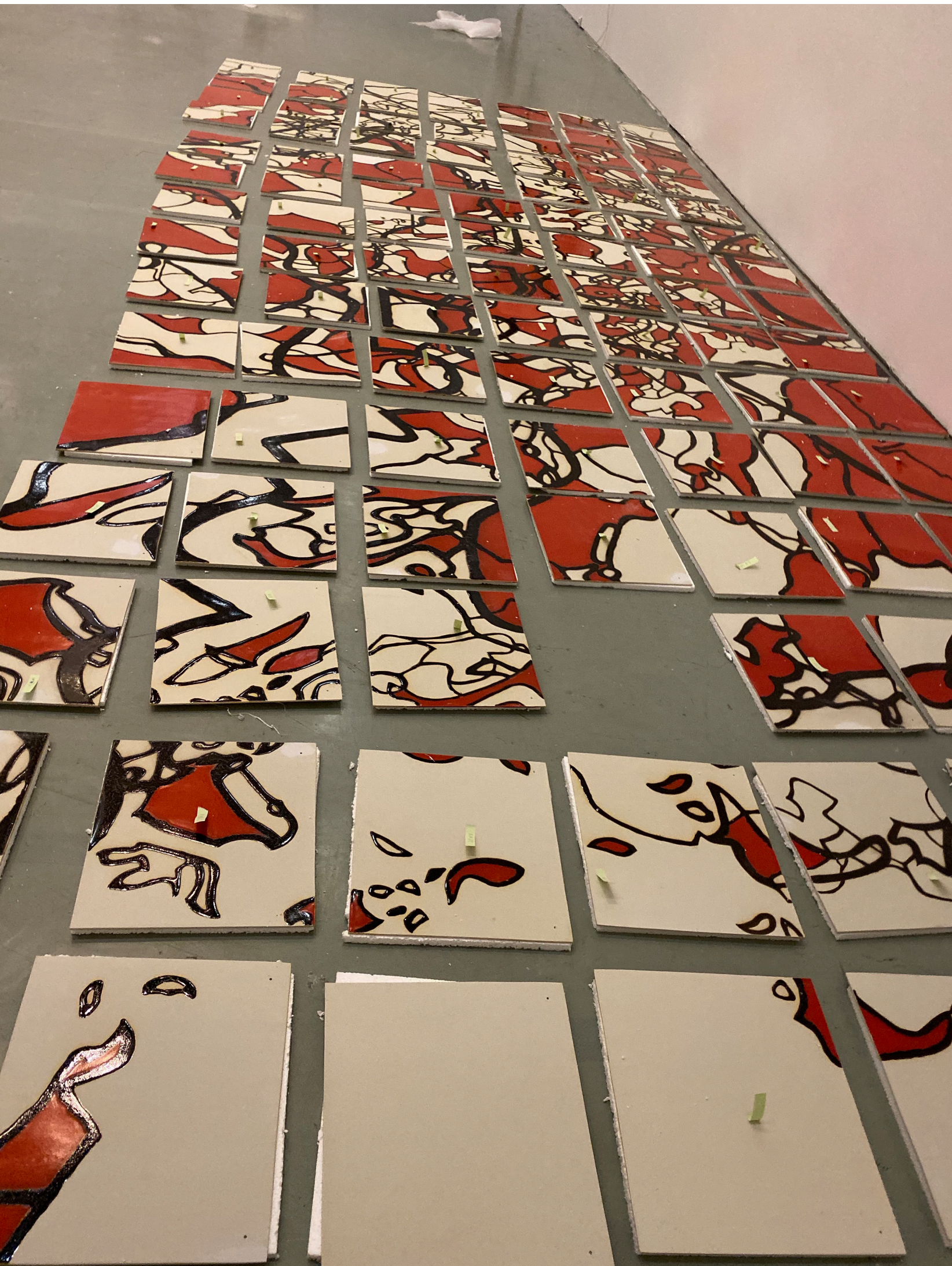
Tiles awaiting installation
