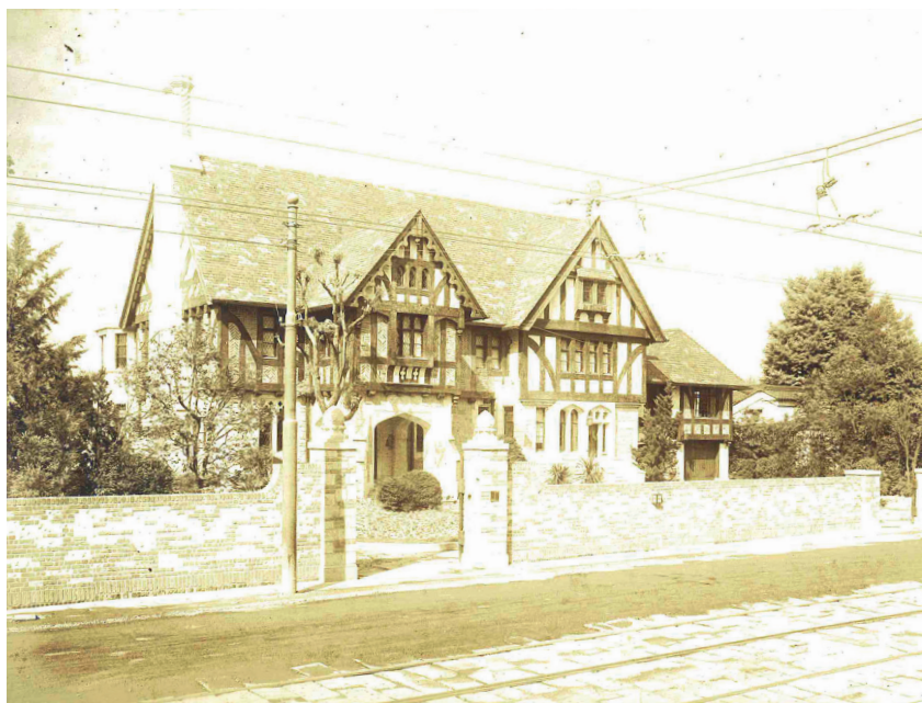
32 Unknown photographer, front elevation from the opposite side of Karasuma Street, Kyoto, 1935, from a presentation album of photographs (upper figure) of the 'Tudor House' designed for Shotaro Shimomura given 'to my friend Bernard Leach'. Crafts Study Centre, ABL/6/2.
