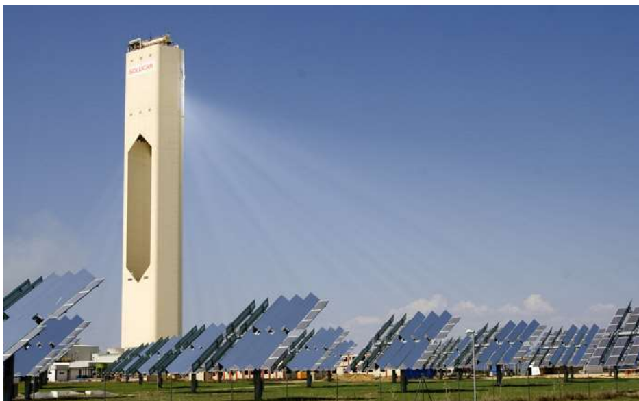
Fig. 8.14. PS-10 Plant, Sevilla, Spain (2007)
