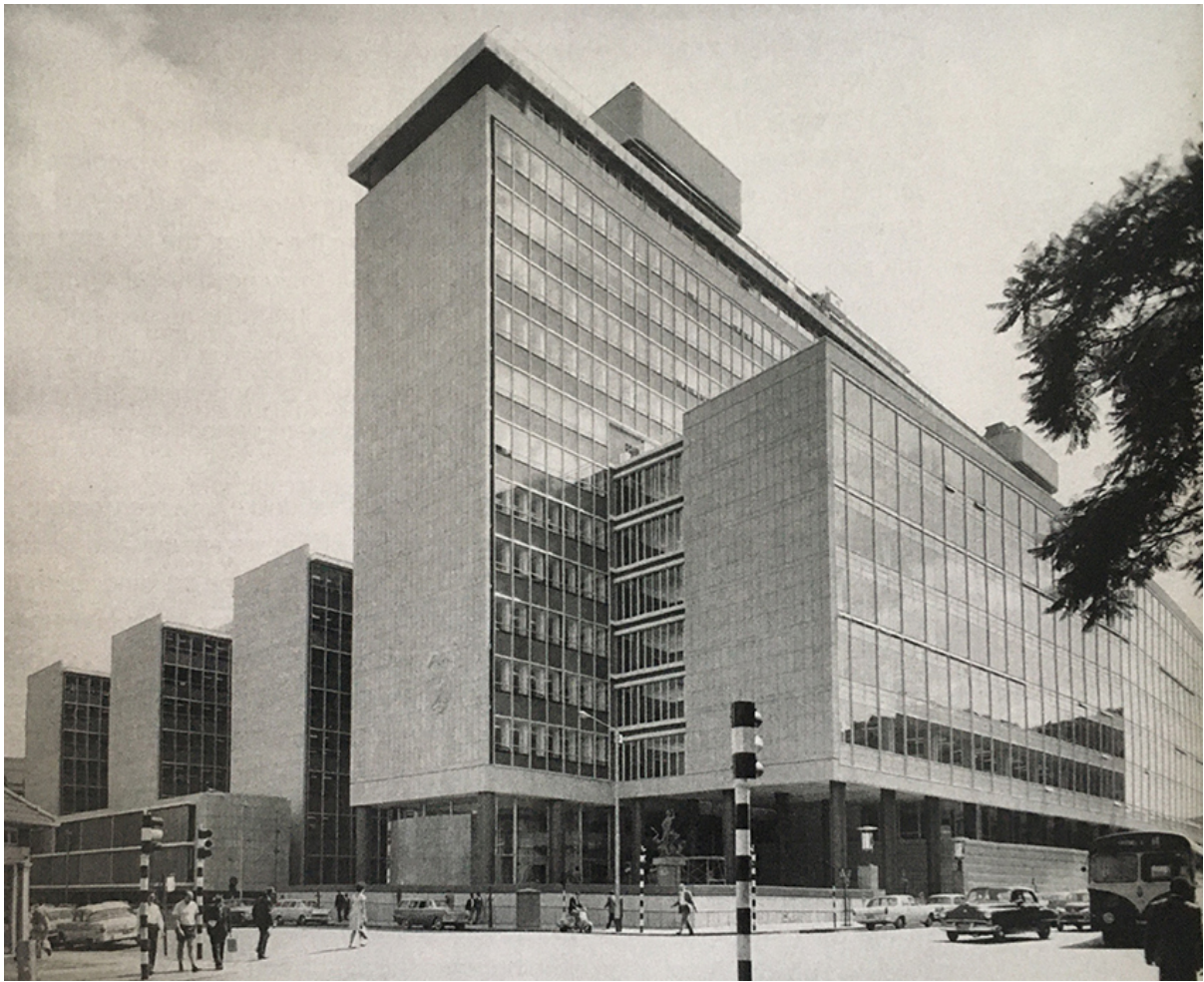
Figure 62. The Transvaal Provincial Administration Building, Pretoria 1962. Architects Moerdyk and Watson, Meiring and Naudé. Dotman Pretorius Photographic Collection, Ditsong National Cultural Museum. Photo credit: Dotman Pretorius.
