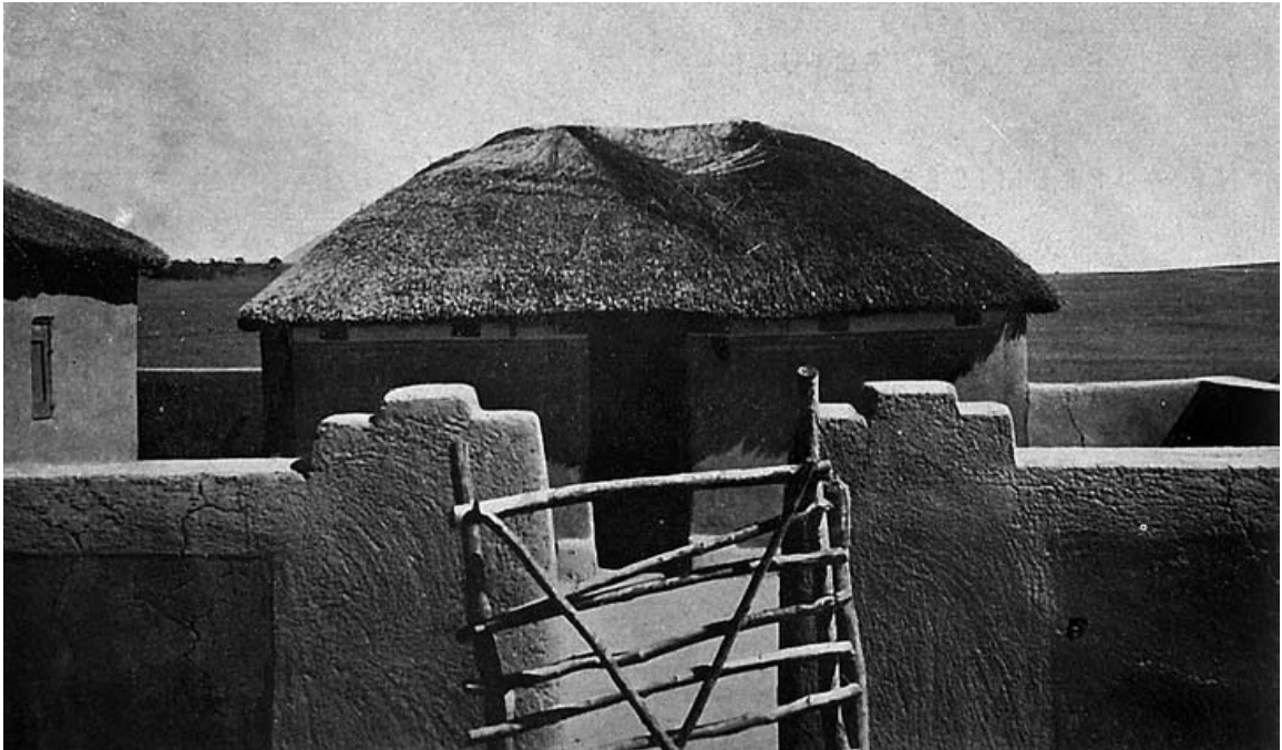
Figure 94. A square on plan Ndebele Chiefs Hut with murals circa 1940. Approximately 22.5 km from Johannesburg. Leading article; 'Native Housing' by Betty Spence. November 1940, South African Architectural Record , Vol. 25, No. 11.
