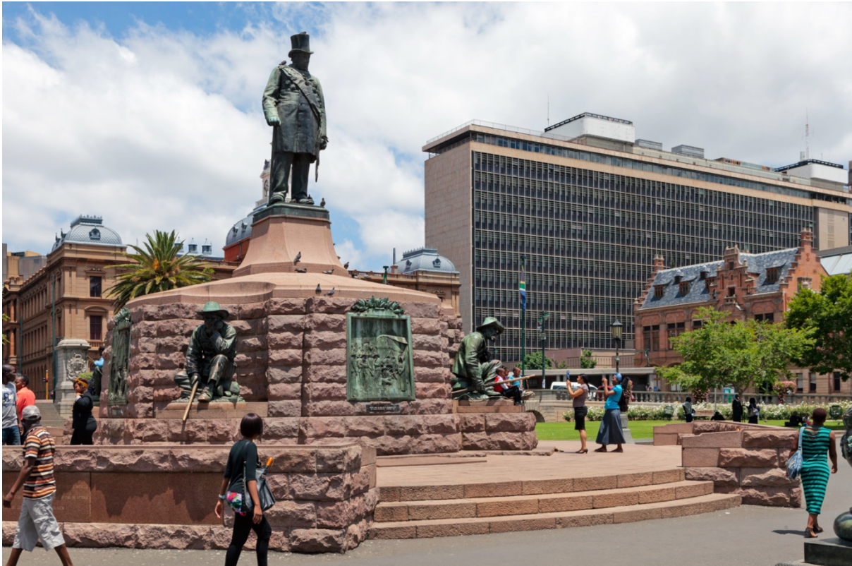
Figure 3. In the background is the abandoned Modernist Transvaal Provincial Administration Building in Pretoria, viewed from Church Square in 2012. Architect team led by A.L. Meiring 1962. In the foreground is the statue of Paul Kruger surrounded by prominent Voortrekker leaders. To the left (partially obscured) is the Raadsaal (Old Council Chambers) 1891, designed by Dutch architect Sytze Wierda in a Renaissance Revival Style. Visible to the right is the Netherlands Bank of South Africa 1897, designed by Dutch architect Willem de Zwaan, and built in Jugendstil, a version of German Art Nouveau. A succession of other colonial styles are present, notably amongst others (not visible here) are Tudor Chambers 1904 designed by George Heys and Herbert Baker's stone fortress-like Reserve Bank in a Classical Revival style completed in 1930. iStock, Photo credit: THEGIFT777.
