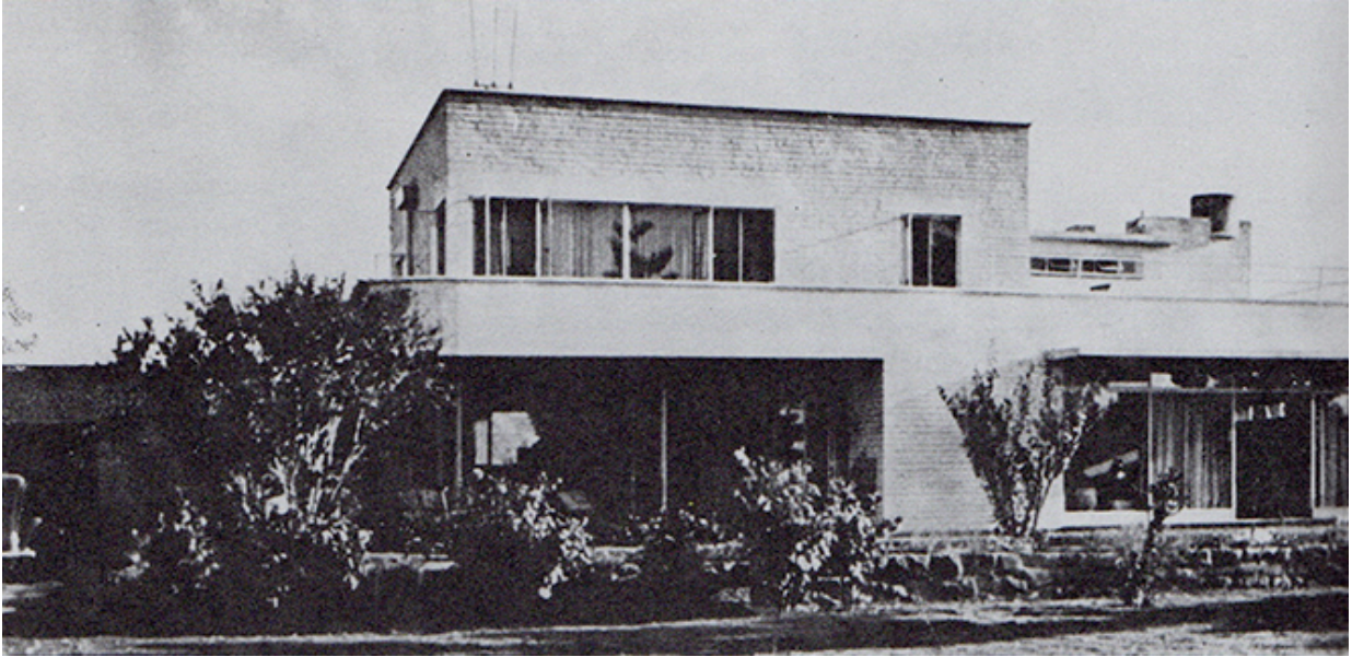
Figure 58. Third Vernacular, House in Brooklyn Pretoria, 1936–37. Architect: W. Gordon McIntosh.
