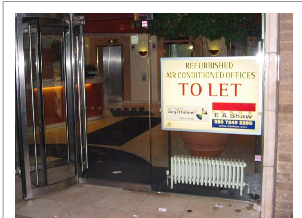
Refurbished Office, London, 2006
